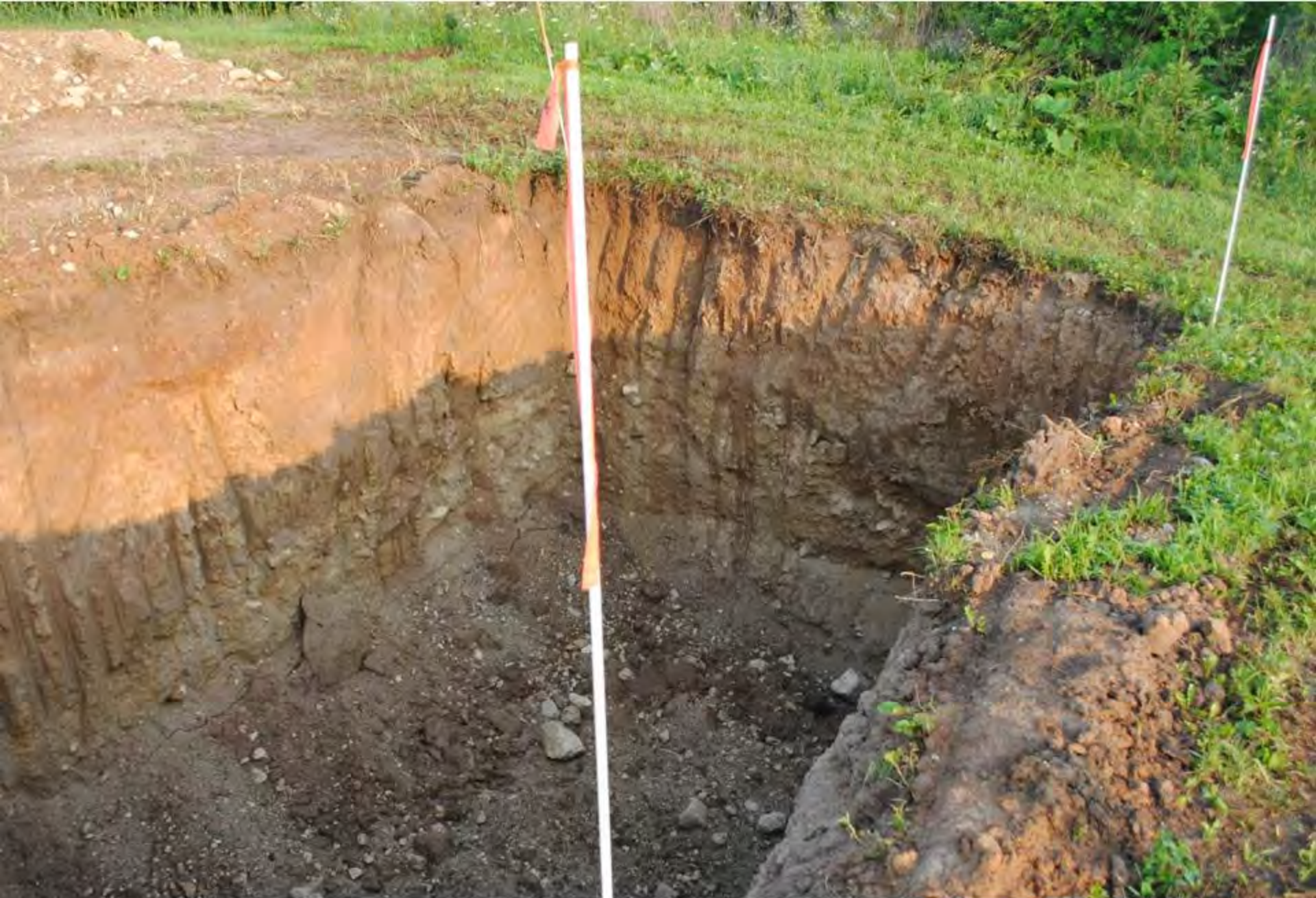
Move earth in preparation of building construction
