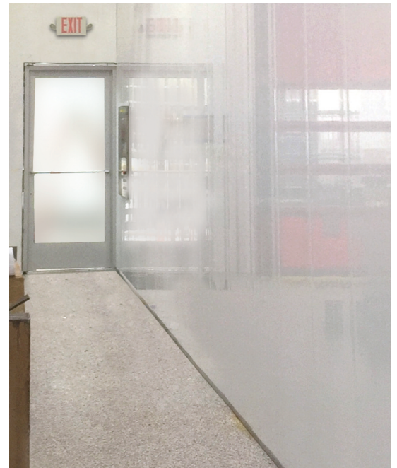
2-1/4" P224 Partition Wall Installation
