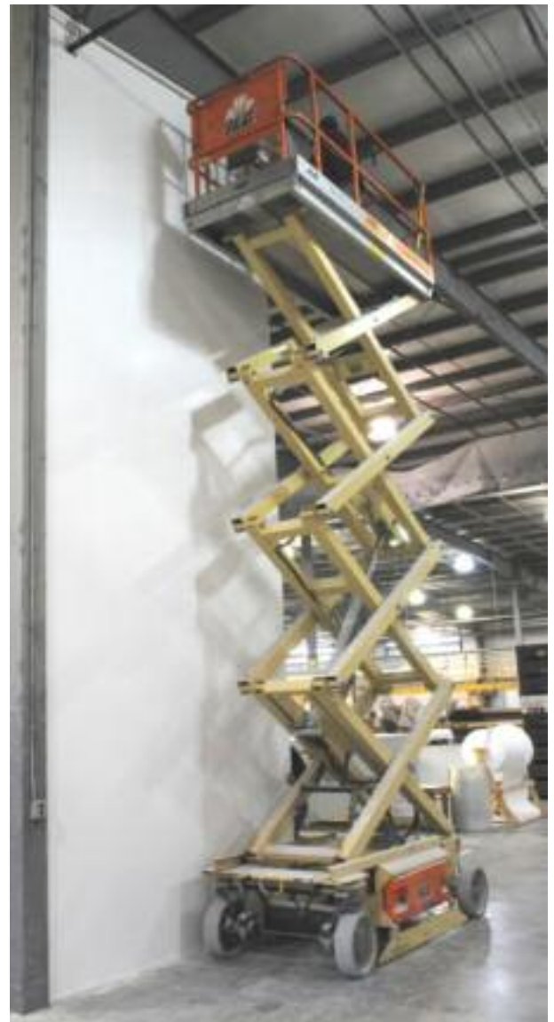
24 Foot High Partition Wall Installation
