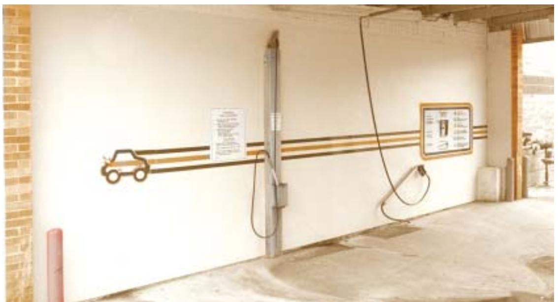
He used rivets only (no adhesive) to mount his panels. Ross said, "they're a little loose and flexible in places, but I like that because we get so much ice in cold weather. All I have to do it hit the panels and since they're a bit flexible the ice cracks and falls right off."
