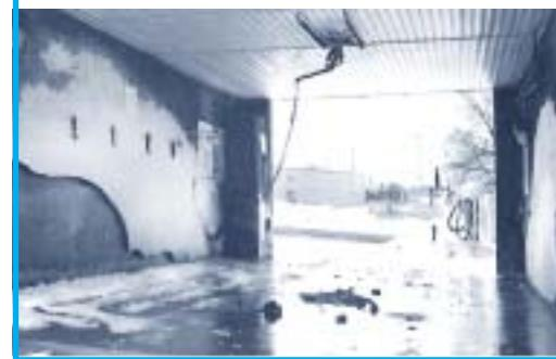
quick enough and on a warm day a huge sheet of ice fell off the wall and landed on the side of a car. It did over \$1600 damage to the car. The \$1600 would have paid to install two bays worth of FRP. With FRP you can just slap the wall with your hand and a small thin sheet of ice falls off with no fuss".
