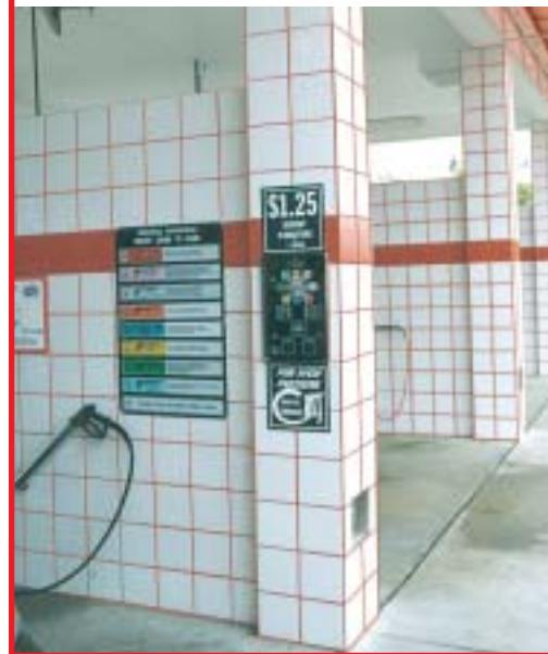
by Frey's company. He uses colored epoxy resin grout that matches the accent tile in the bay. By using the colored grout, it prevents the dirt from showing easily. The tile they use is a fired ceramic tile usually 8 x 8, but recently they have been using larger 10 x 10 or even 12 x 12 tiles. Greg recommends using Klean Wall (see info under Spray-on Fiberglass for more detail), a mild acid cleaner to prevent etching of the tile.
