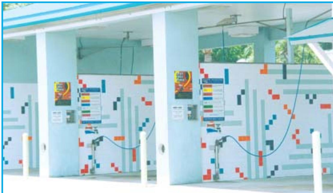
Here's a wash (Pronto Wash in St. Petersburg) that demonstrates an especially colorful and rather “artsy”, free spirited use of tile in its SS bays. The “eclectic” design/layout of tile in diverse colors tends to be a bit more forgiving of overspray stain and makes for less noticeable replacement of any broken tiles.
