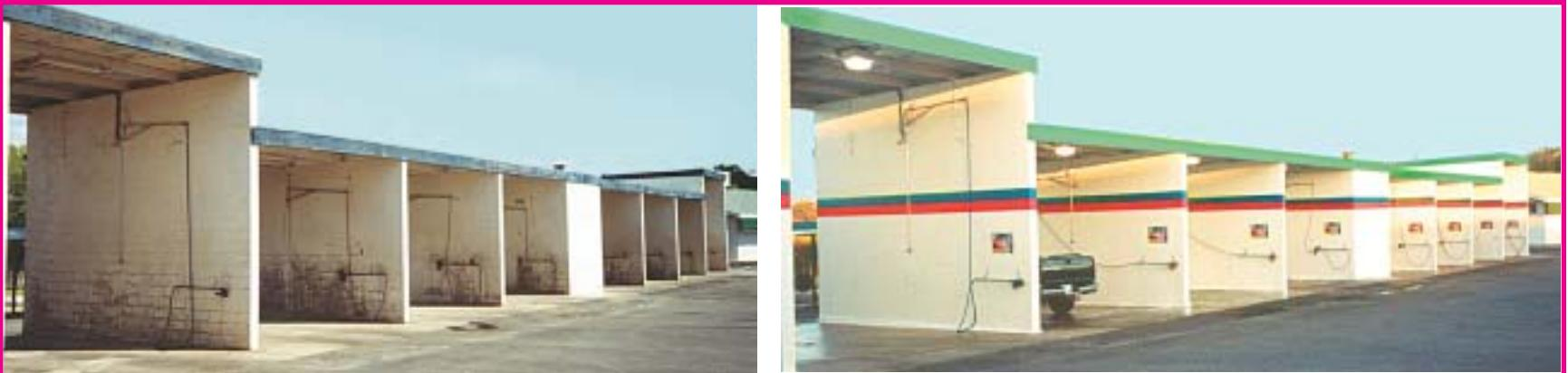
Bill Sartor transformed the walls of this tired ol' grungy 8 bay in San Antone via spray-on fiberglass. The result: bright, slick, durable, easy to clean/maintain walls that incorporate a sharp, lively blue and red "racing stripe" as an integral part of the wall coating.
