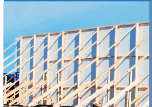
Typical bracing installation of Extrutech FORM™ Wall – a 17 ft x 50 ft area shown.
