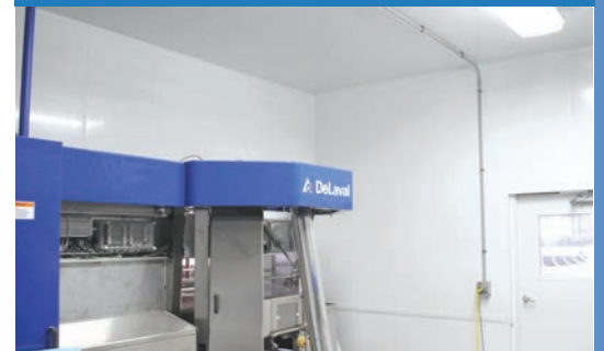
Interior of Robotic Room Walls
