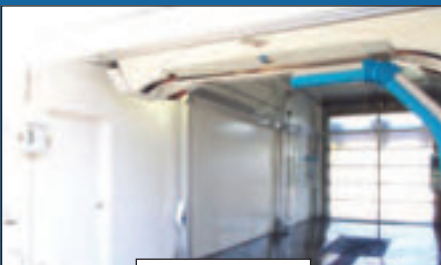
Car Wash Walls
