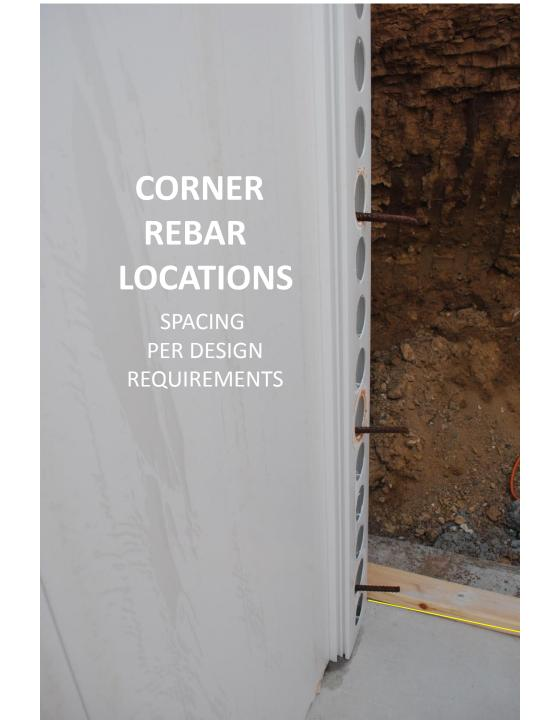
Install FORM Panels by tipping bottom edges into installed panel and bushing top into place until seams are touching.
